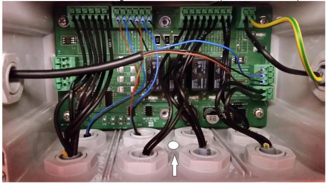
3. The wire must be laid and shaped as shown in the picture, it should bend before entering the box. Then all the water will be directed away from the box. Loosen all the straps attached to the hydraulic hoses.
